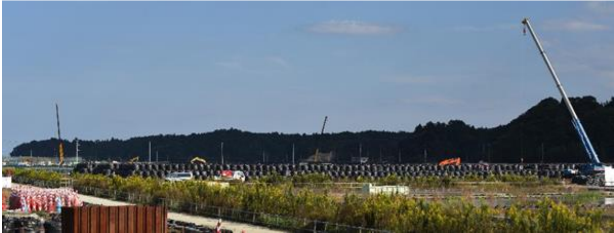
Figure 2. A bale storage site mid-construction, aiming to concentrate contamination.
