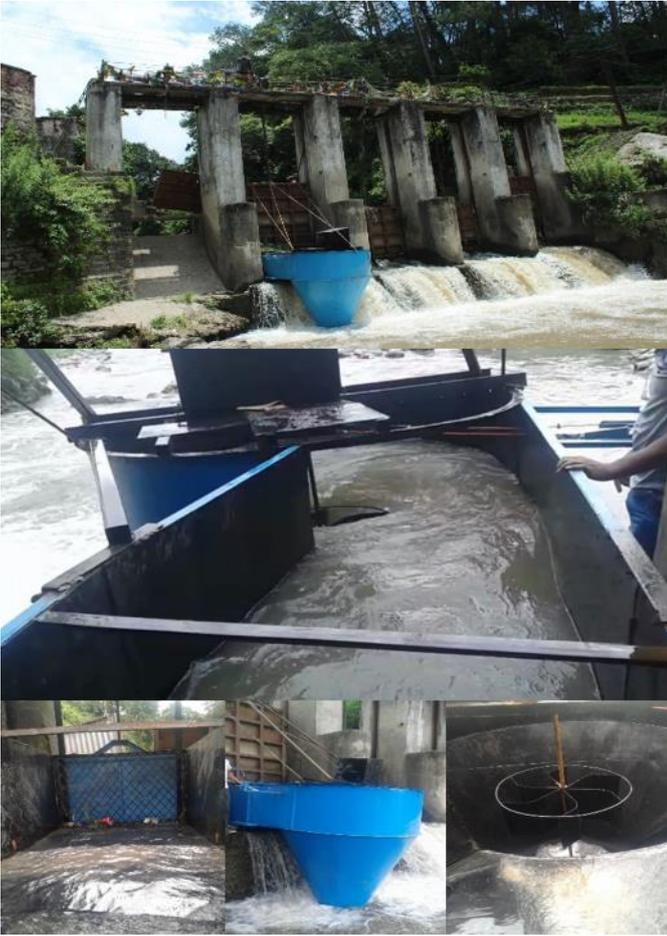
Figure 5. Pilot project using conical basin structure, with integration in irrigation canal weir, intake canal, basin structure and runner.
