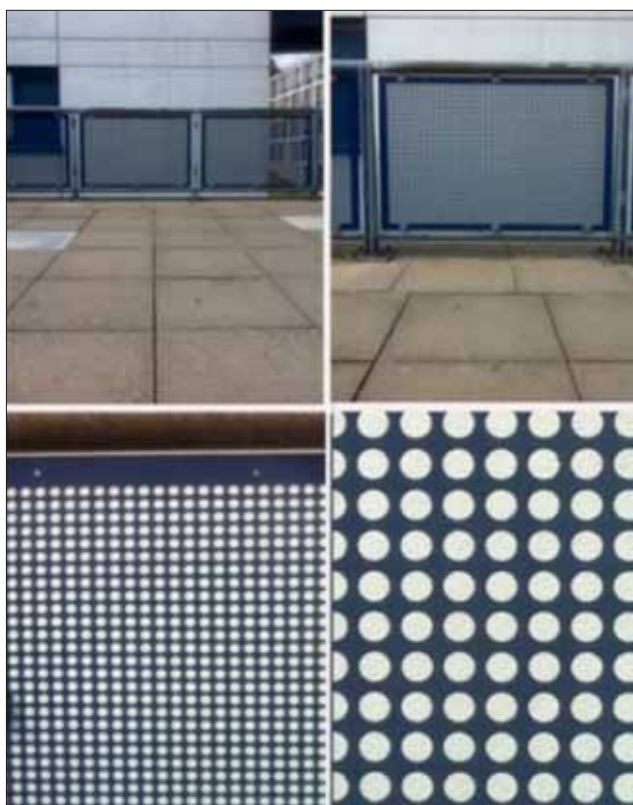
Figure 4. A pattern on railings photographed at various distances to show how the effects of pattern size and spatial frequency combine to determine discomfort.
