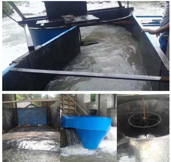
Fig. 16: Pilot Project using conical basin structure (canal, gate, basin structure and runner)
