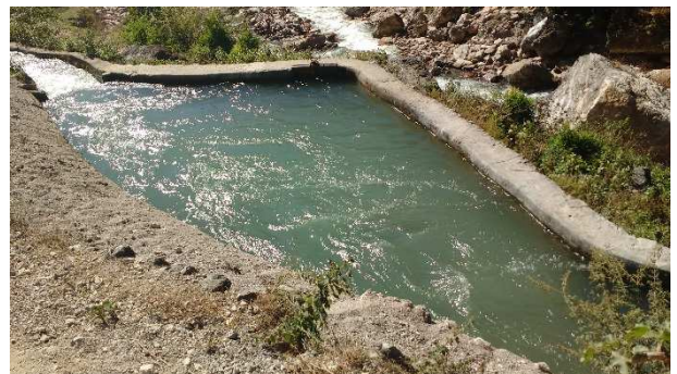
Fig. 5. Ineffective shape of desilting bay
