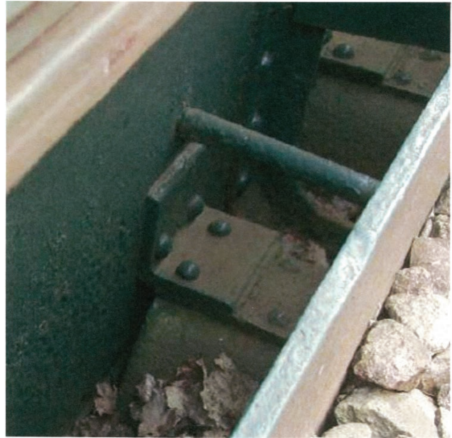
Figure 5. Tie bar above trough deck level
